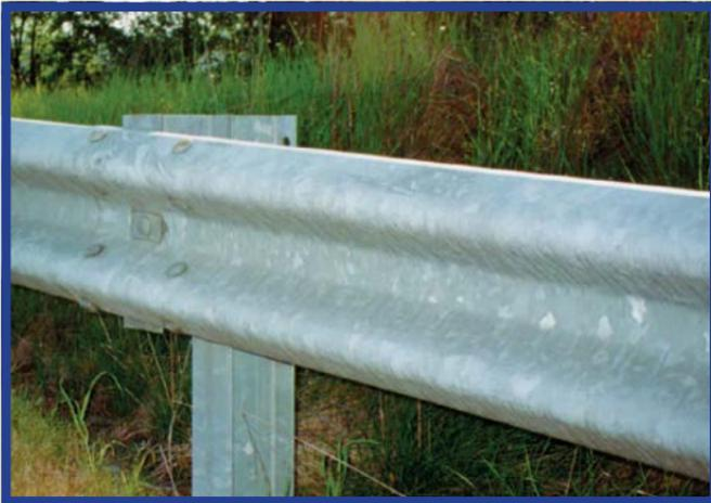
***The zinc patina on a piece of fully weathered steel, seen left, will create a more successful duplex system when left on the surface.***
