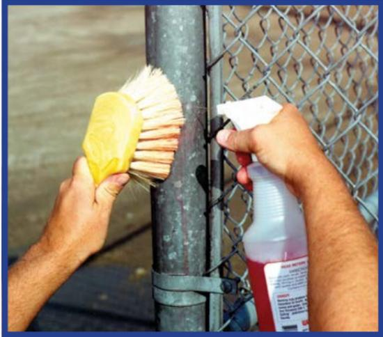
*Organic contaminants can be removed using alkaline or acidic solutions, or solvent cleaning.*
